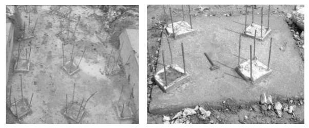
Figure 1 – Square piles turning around its axis by 45° during pilling
