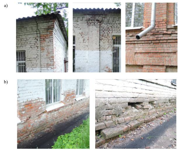
Figure 2 – Atmospheric moisture effects to brickwork of buildings enclosing structures:
